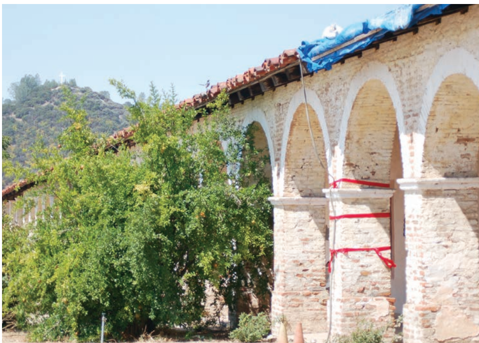
View of South Convento, looking to the West. This is the area that will be addressed next in the progression of five Phases.
