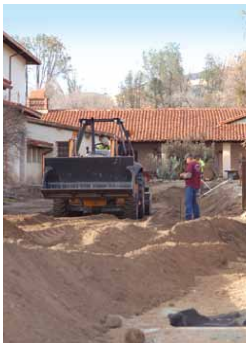
Grading of the east side of the church and installation of proper drainage.
