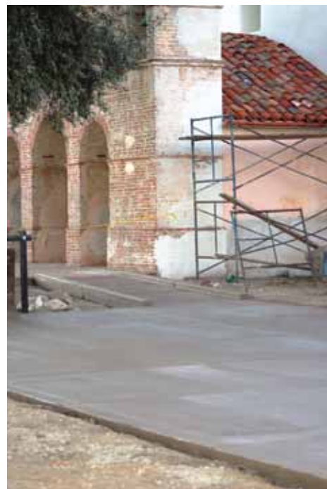
Installation of the handicap parking area and ADA compliant ramp at the entrance area of the church.
