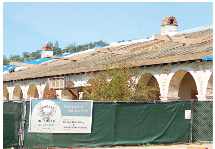
Construction continues on the south convento.
