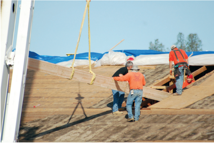
The construction crew installs roof beams on the south convento.
