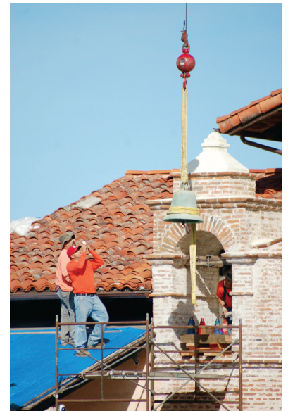
Workers watch as a crane carefully removes the damaged bell.
