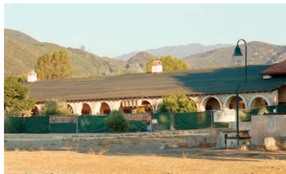
The roof prepped for the installation of the new clay tiles.
