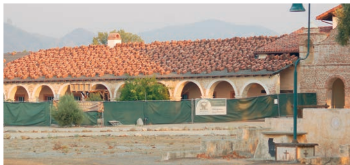
Tile installation in progress.
