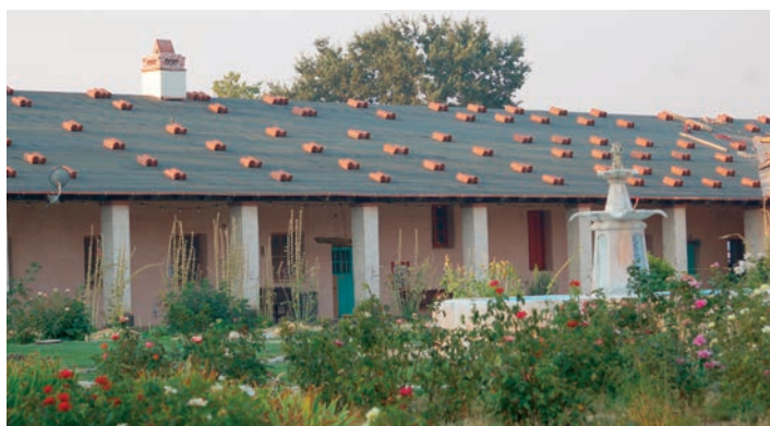
The clay tiles are stacked ready to be installed.
