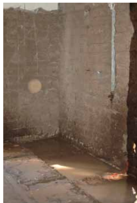
West Convento shower, reduced back to original adobe wall to facilitate new plumbing.
