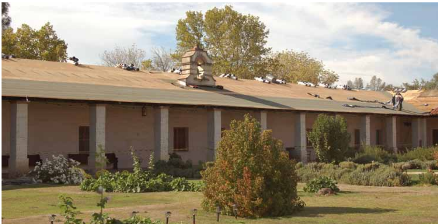
Western Convento roof receiving under layment in preparation for return of roofing tiles.
