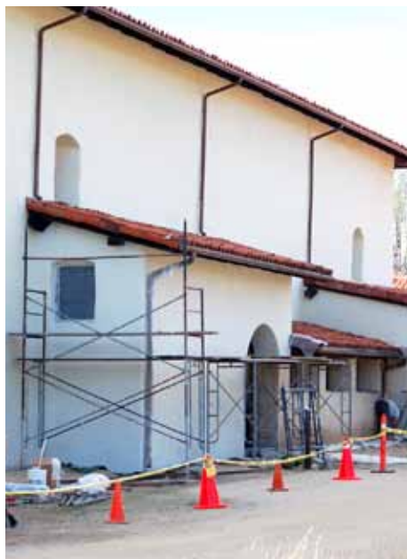
Outside eastern wall of the church, Baptistry and St. Anthony room exteriors walls are being lime washed to match the rest of the exterior church walls.
