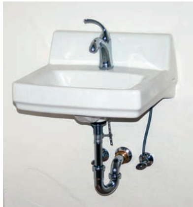
New plumbing/sinks have been installed in private retreat rooms by Knecht Plumbing and Heating.
