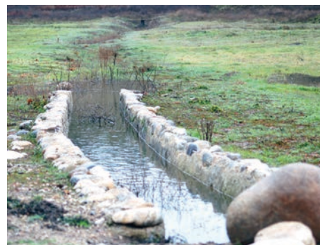
The old Mission aqueduct is still on duty, moving water across the acres of Mission grounds for use in tannery, grist mill and irrigating crops.
