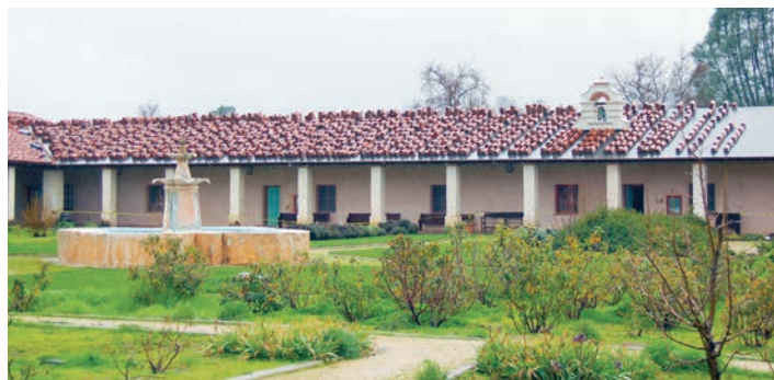
Tiles returning to the roof of the West Convento, courtesy of Nieporte Roofing.
