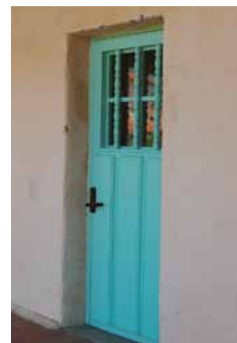
All external Convento doors will now share this fresh color.
