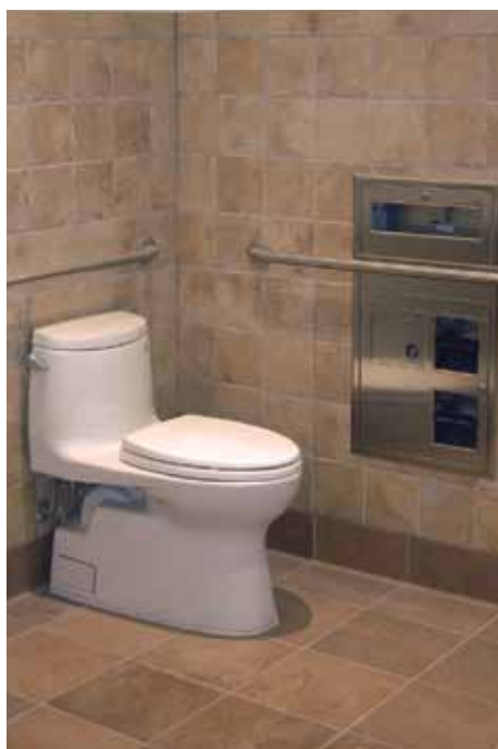
New bathroom in the West Convento retreat wing.
