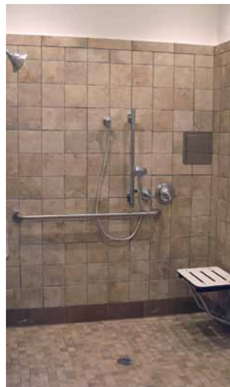
New ADA compliant shower in west wing.
