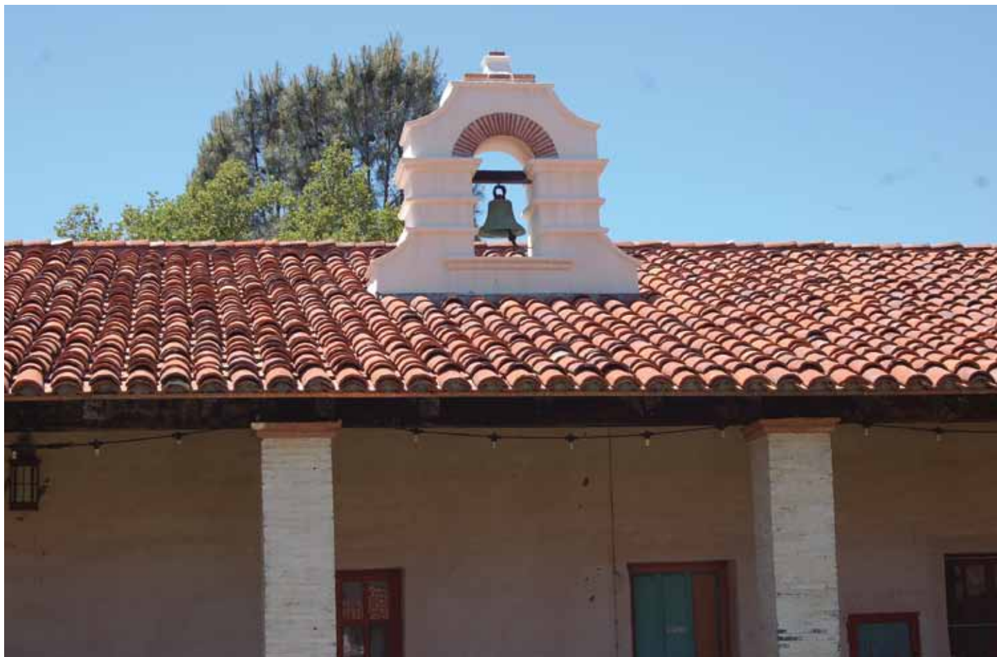
West Convento roof once again has its tile covering.
