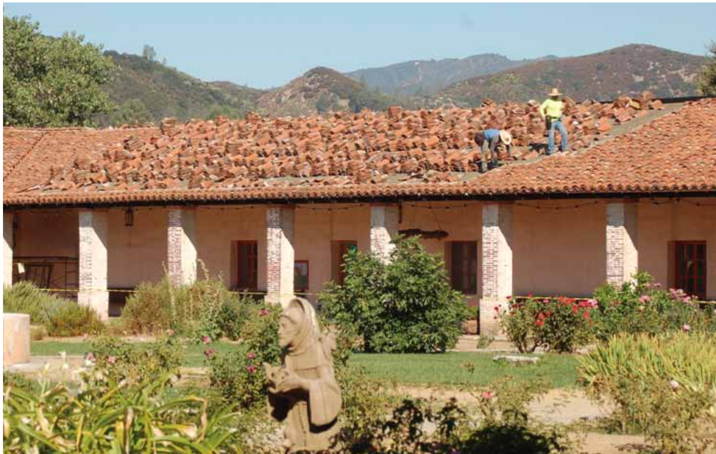
North Convento roofing tiles being replaced after completion of seismic work on this wing.
