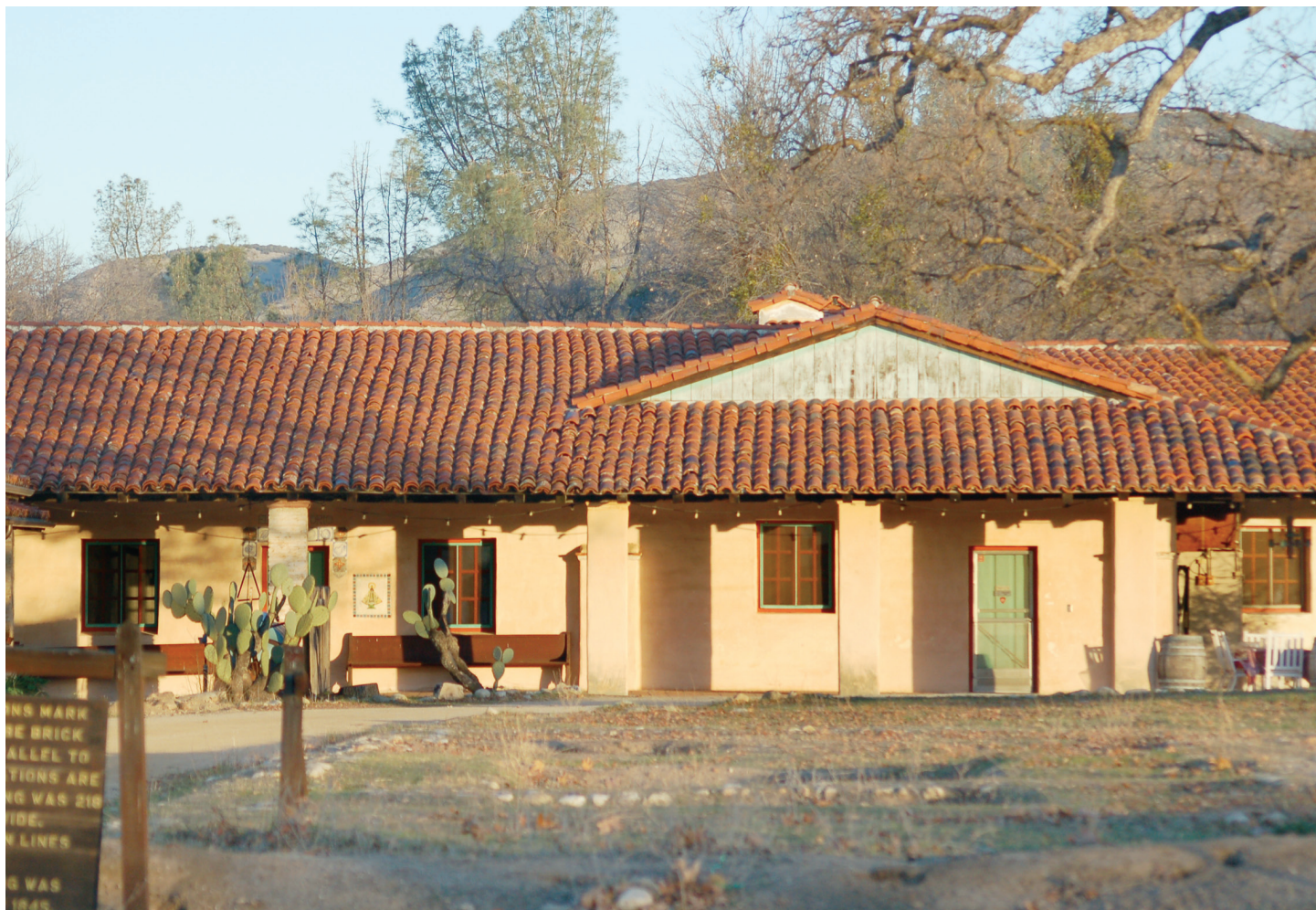
Phase V includes the northeast wing of the Mission complex from the dining rooms through to the stables.
