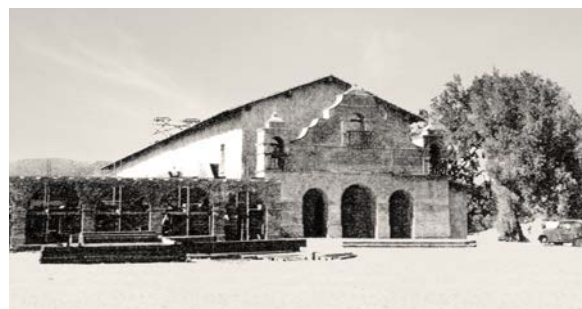
View north of church and part of Convento during construction, ca. 1949 (image from Mission San Antonio Archives)
