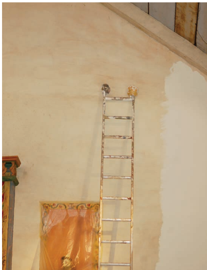
Pete Vachek has done an amazing job painting the interior of the church.
