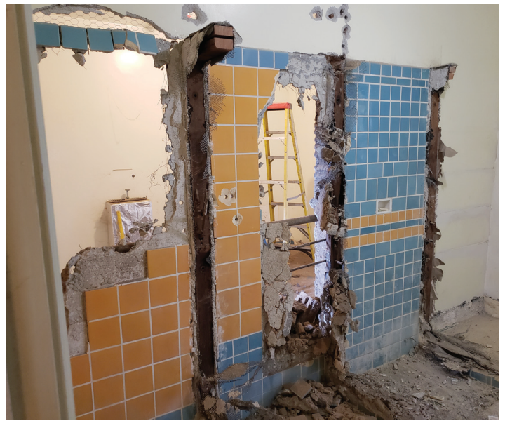
Demolition of walls in North Wing makes way for new ADA compliant bathrooms.
