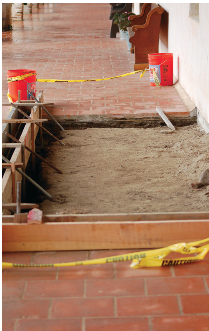
Preparation for new ADA compliant ramps for North Retreat Corridor.
