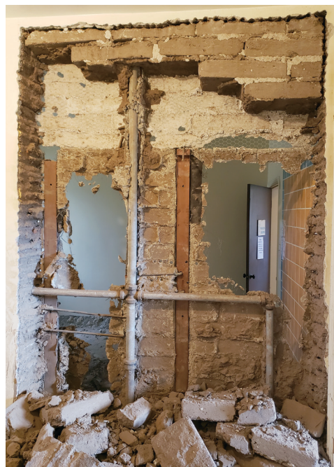
Demolition of walls in North Wing makes way for new ADA compliant bathrooms.
