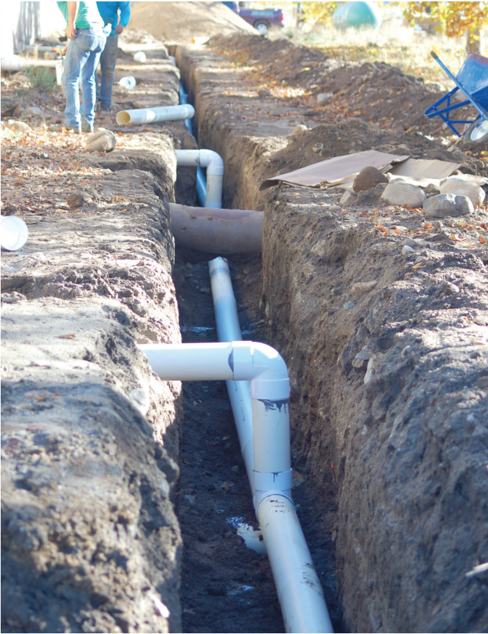
West side of Mission, new drainage system.
