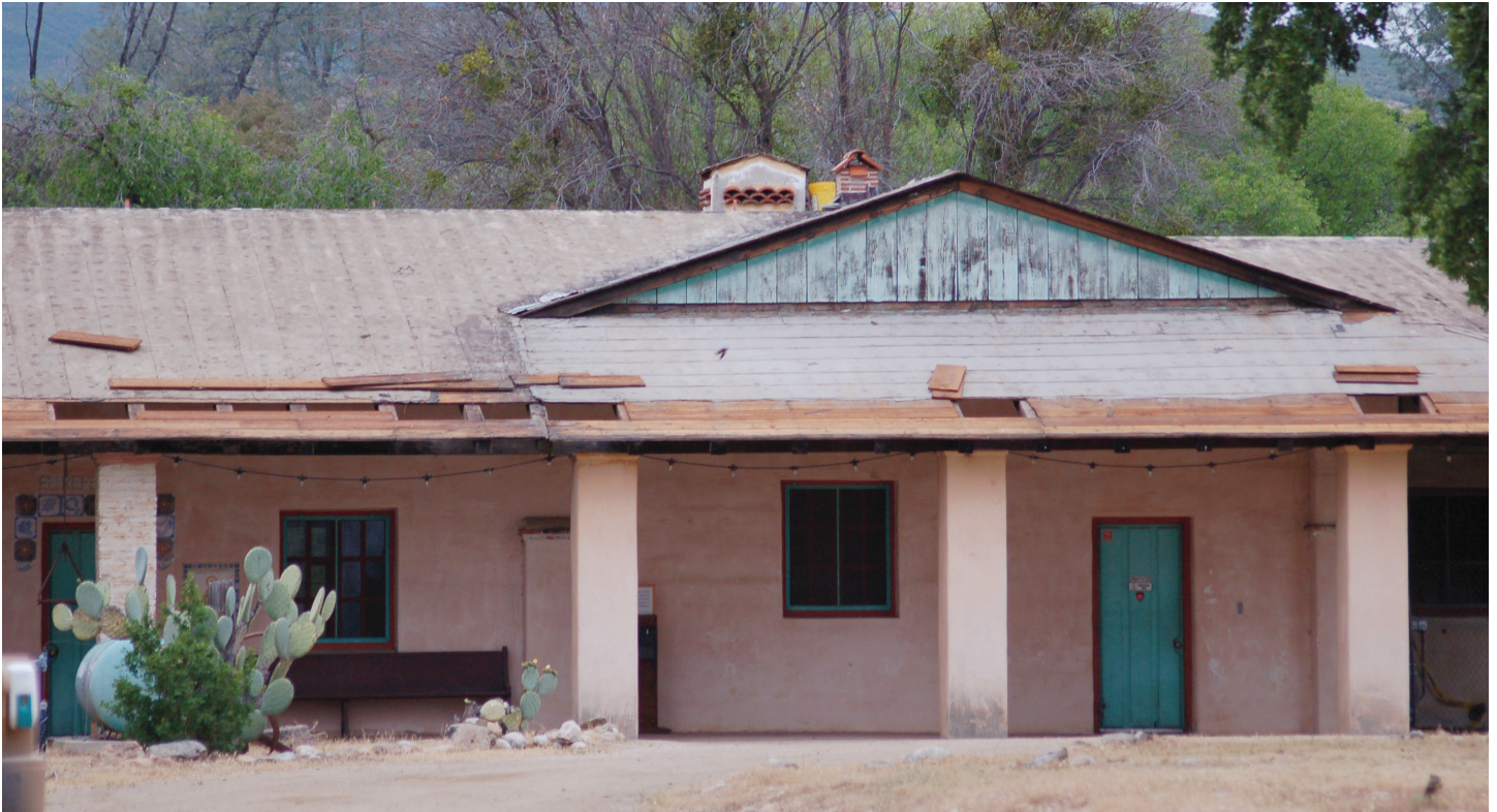
Phase V work begins with the removal of the roofing tile and underlayment on the northeast end of the facilities.
