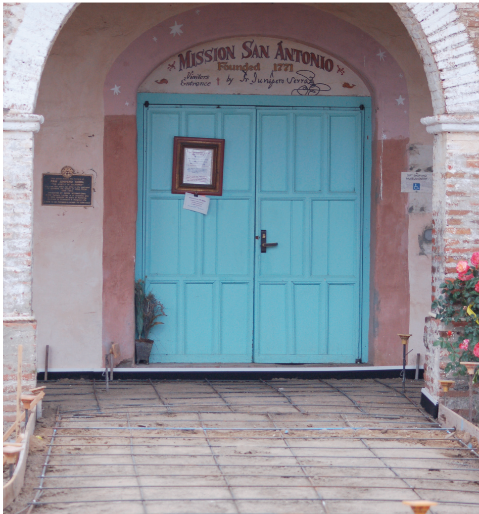
ADA-compliant concrete entry to Gift Shop replaces tile.
