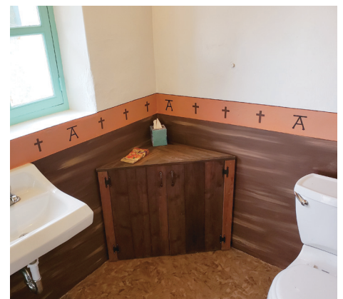
New wainscoting painted on walls of restroom by kitchen by Pete Vachek; new cabinet built by Sean Steele.
