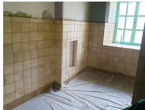
New ADA-compliant bathroom under construction in north retreat wing.
