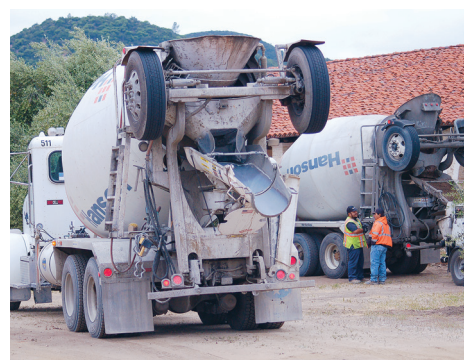
First of the cement trucks arrive to begin pouring the concrete.
