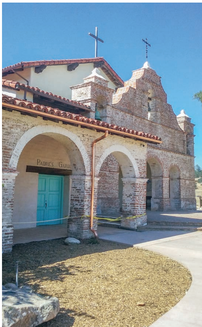
New copper gutters have been installed on the South exposure of Mission.
