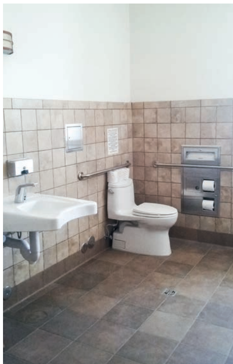
New ADA compliant restroom in North Retreat Wing.
