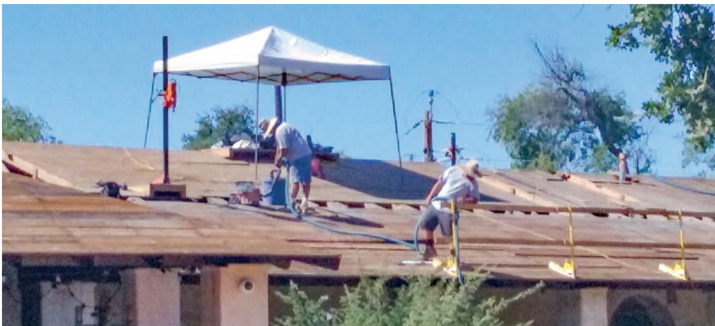
Work on Phase 5 is definitely Hot!
