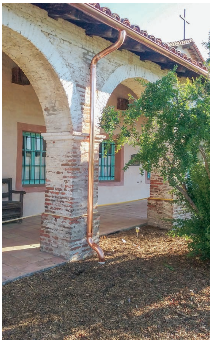
New copper gutters have been installed on the South exposure of Mission.
