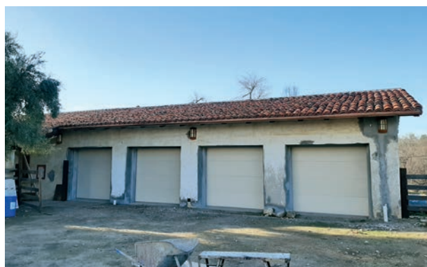
New garage doors and lighting—northeast wing.
