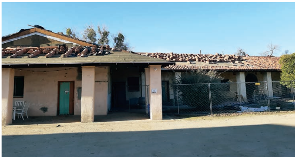
Roofing tiles going back onto roof, signaling conclusion of seismic stabilization work.
