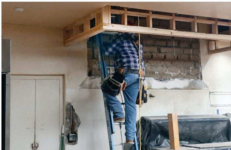
Not Santa...just Bill working on framing for new kitchen hood.
