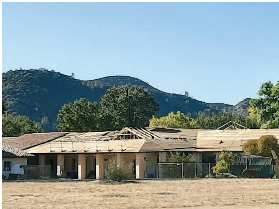
Northeast wing roofing tiles removed to let seismic work commence.
