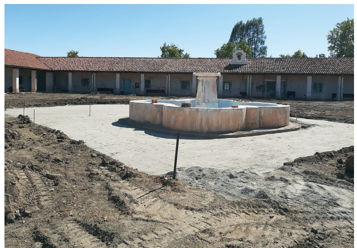
Fountain repair process has begun. Brush Concrete (via Mark Switzer Excavating) begins hardscape August 3, 2020.
