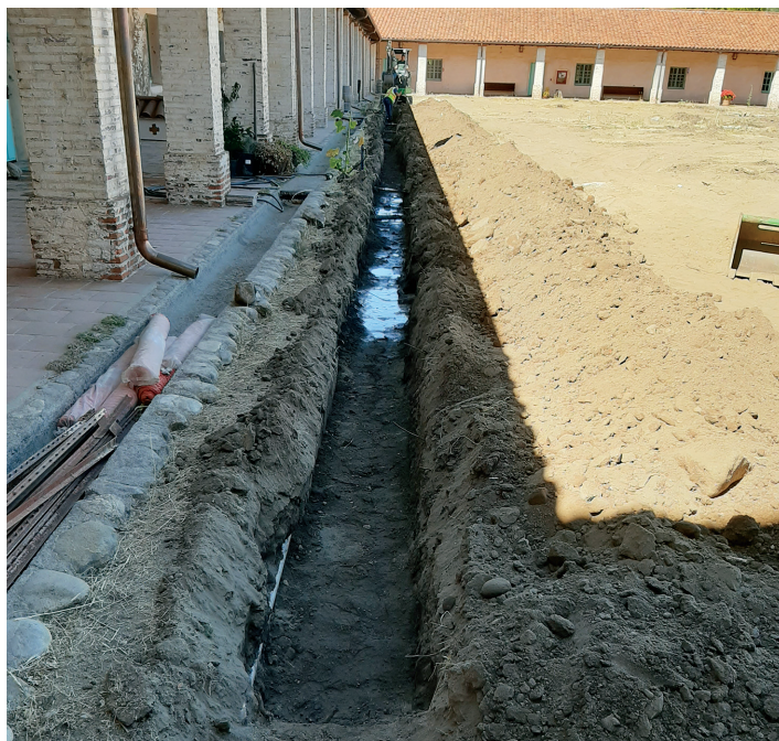
New water lines replace old deteriorating one in quadrangle's Padres' Garden.
