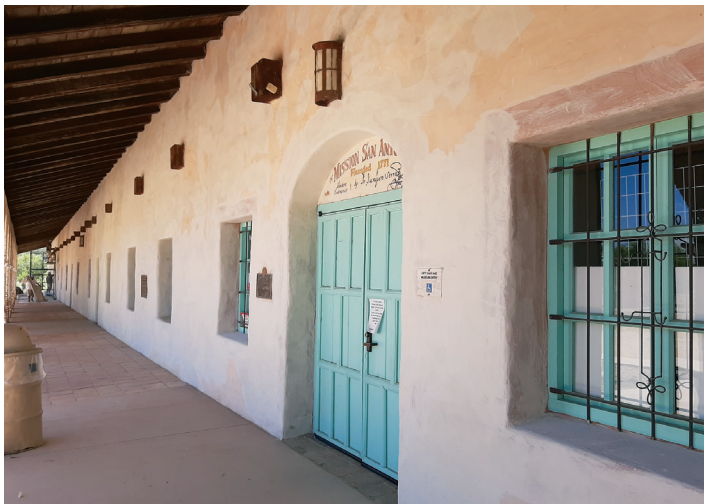
Front (South) external corridor nears completion of the fabric repair and limewash.
