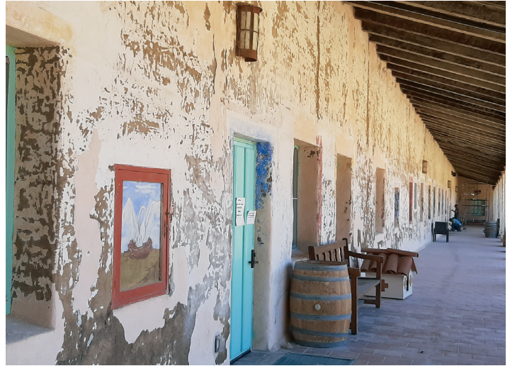
South exterior wall located in quadrangle amid fabric repair process.
