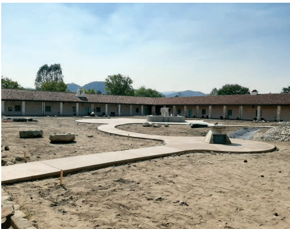
Garden pathway poured.
