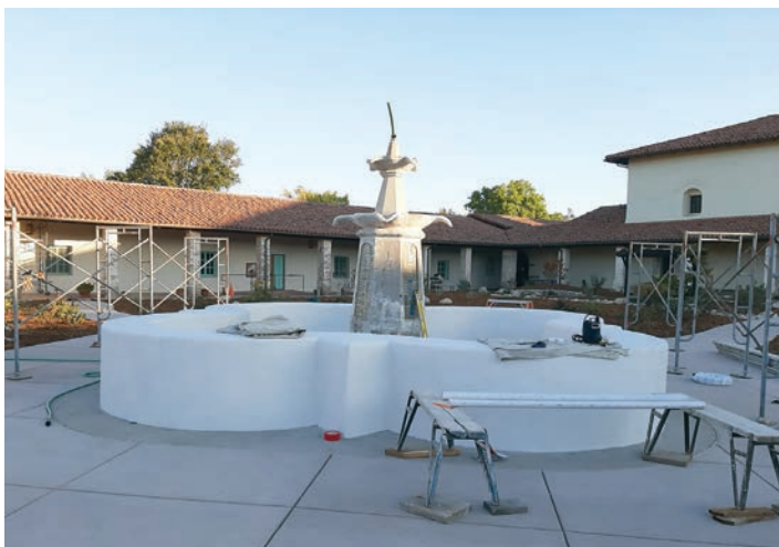
Foundation restoration in progress.
