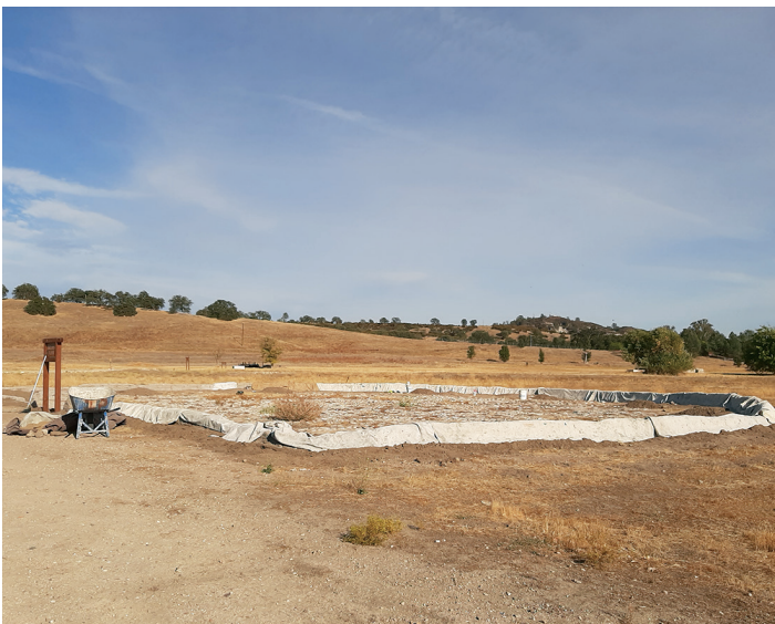
Stabilization and preservation of the threshing floor
