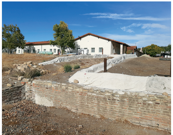
Stabilization and preservation of the ruin walls of the Lavandaria
