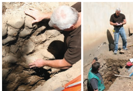
Exterior Test Pits excavated by the Geologist on the East side of the church in order to ascertain foundation depth and material, soils composition, water table, etc.
