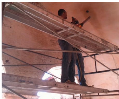
Test cores being taken by ARG in the vault behind the Campanario to determine material (concrete here), quality, etc. The holes were then patched with a compatible material.
