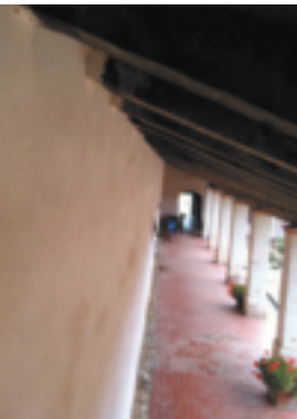
Birds eye view of how the loggia rafters pocket into the church walls
