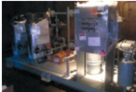
Newly arrived boiler
