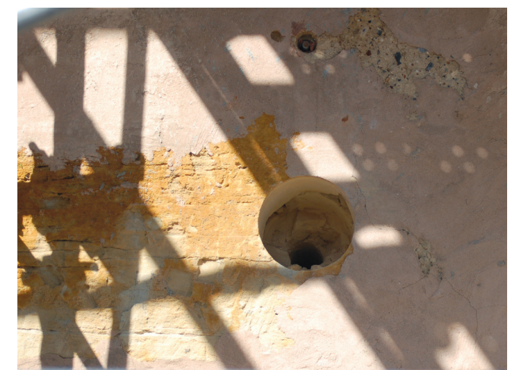
Restoration work in progress at Carmel Mission
